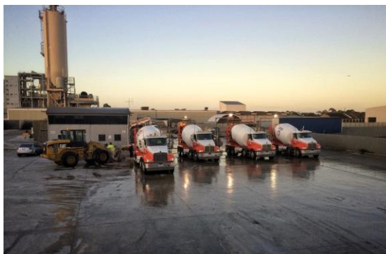
Central Campbellfield site
